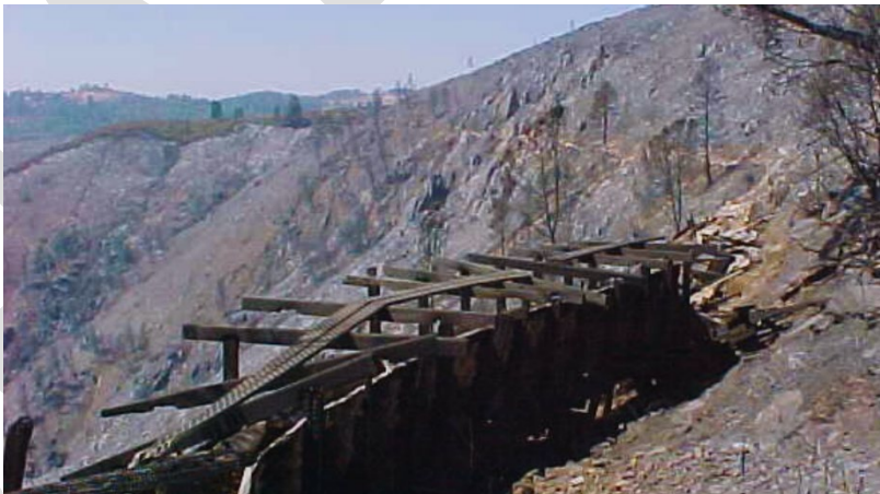
Figure 8. Three-Quarter mile flume destroyed by the Darby Fire.
